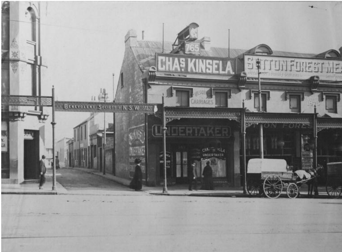
Plate 3.1 North-west view showing Valentine Lane and 761 to 765 George Street in 1910 (NSCA CRS 51/2652).
